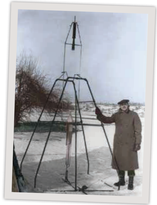
Robert Goddard on March 16, 1926, holding the launch frame for a rocket of his own design.
